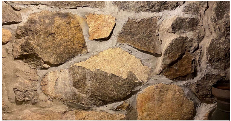
interior rubble foundation wall
