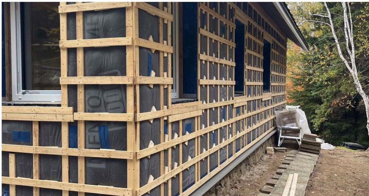
Larson Truss Method, filled with cellulose and prepared for the addition of cedar siding
