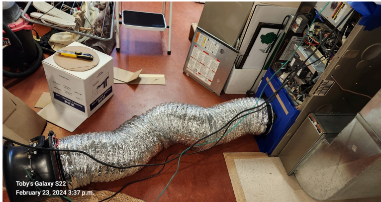
Measuring duct leakage - results inconclusive with this method.
