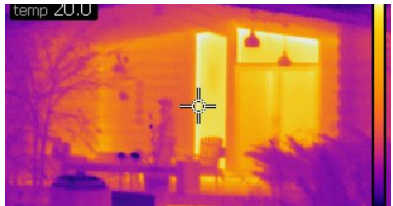
The front door and ceiling heat loss was high
