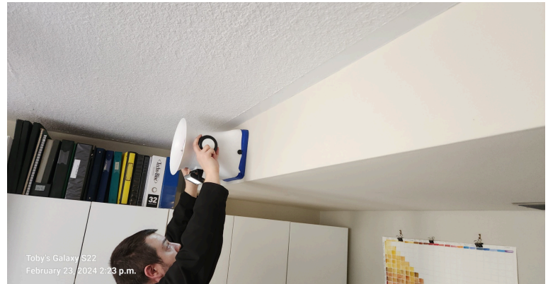
Checking supply duct flow of all registers to estimate leakage.
