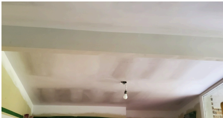
Insulation was added to the cathedral ceiling
