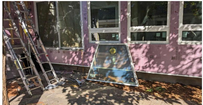
New windows going in
