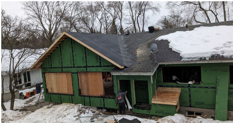
Exterior insulation mid-construction
