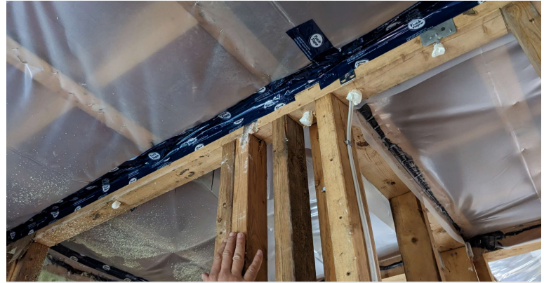
Sealing for insulation
