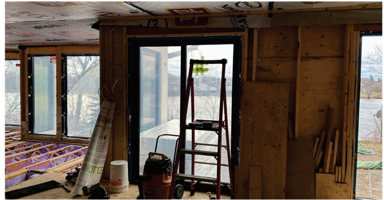
The house was taken down to the studs; added insulation, windows, doors
