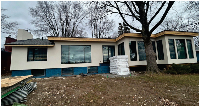
Extensive flat roof construction on river side. All new windows and doors.
