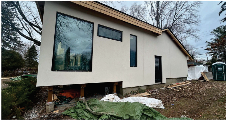
Exterior Insulation and Finish Systems (EIFS) and large windows with river view
