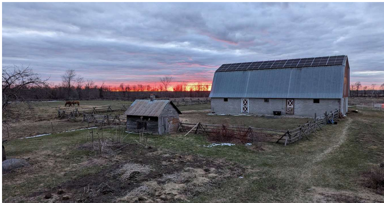
Solar generation on barn - outbuilding
