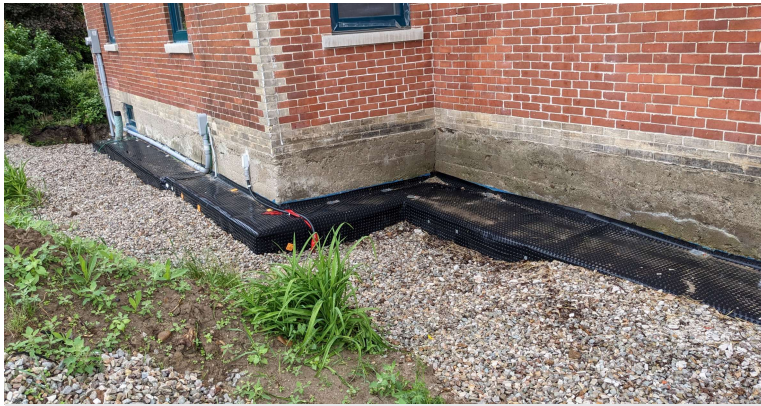
ICF detail reinforcing lower part of foundation
