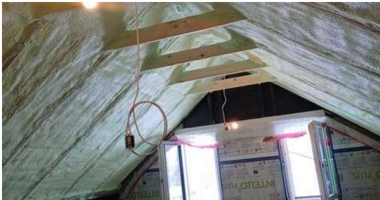
Hot roof detail - rafter cavities cleaned and closed cell spray foam added
