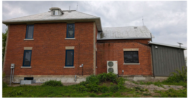
New Windows and new Air Source Heat Pump
