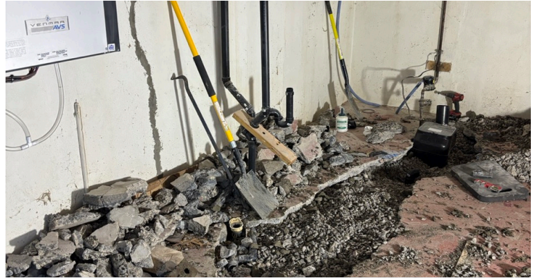
Sub-Slab Plumbing Replacement
