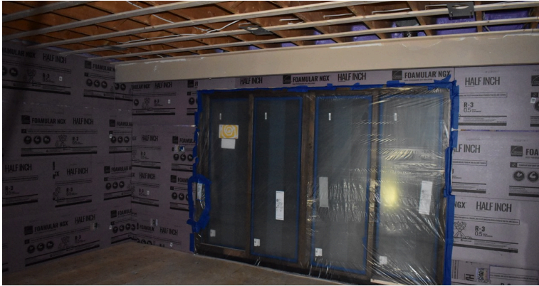
Sliding Door Replacement & New XPS Insulation
