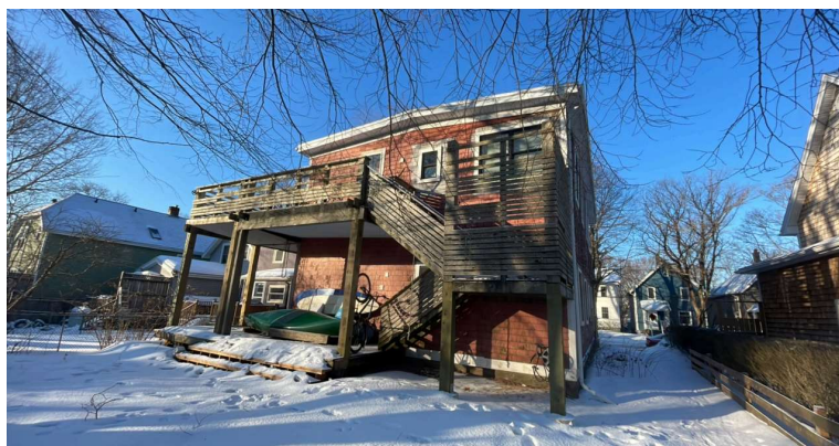
Rear exterior of home with access to upper unit
