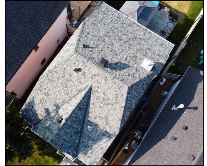
Class 4 IR Roof Cover – Calgary, 2022
