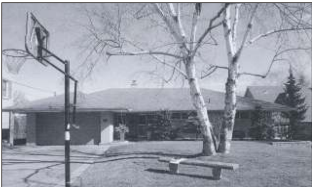
■ Whole House renovation before ...
