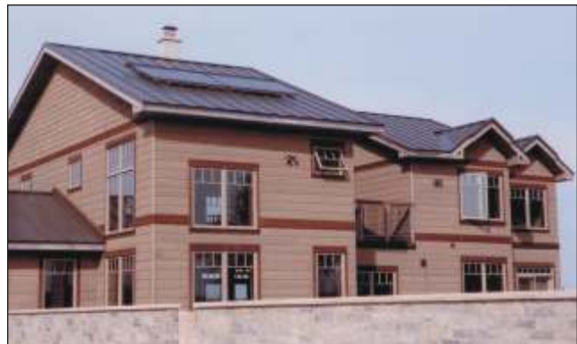
■ FUNCTIONALITY and environmental performance are the earmarks of this residence in Hamilton, Ont. It won the new "Green Home Award" for its developer, New Horizon Homes. The three-bedroom family home provides lots of open, liveable space, and natural light fills every room — an added benefit of passive solar design.
