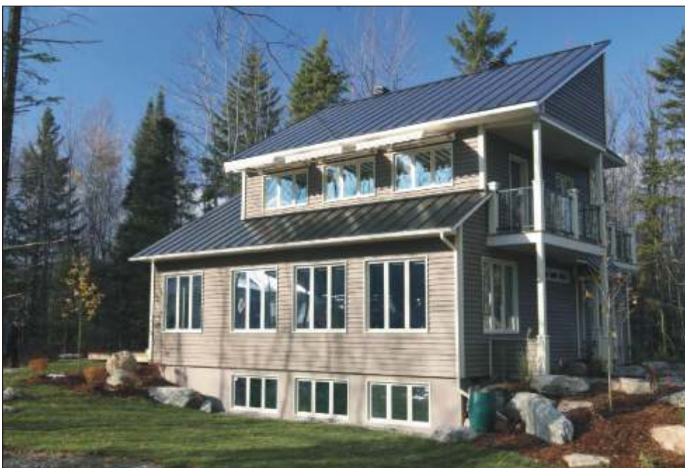
■ ÉCOTERRA EQuilibrium project in Eastman, Que., uses innovative features including solar thermal "harvesting" to achieve net zero energy rating.
