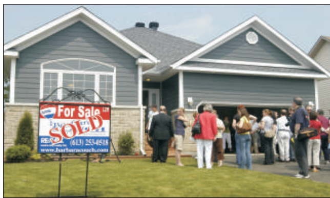
■ HALLIDAY HOMES used 14 students as part of construction team for this EnviroHome in Carleton Place near Ottawa.
