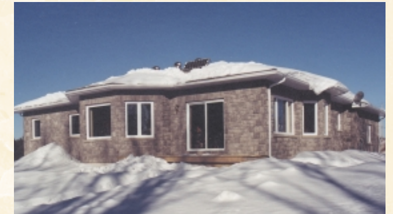
Teixeira EnviroHome, Teixeira Construction Ltd.
