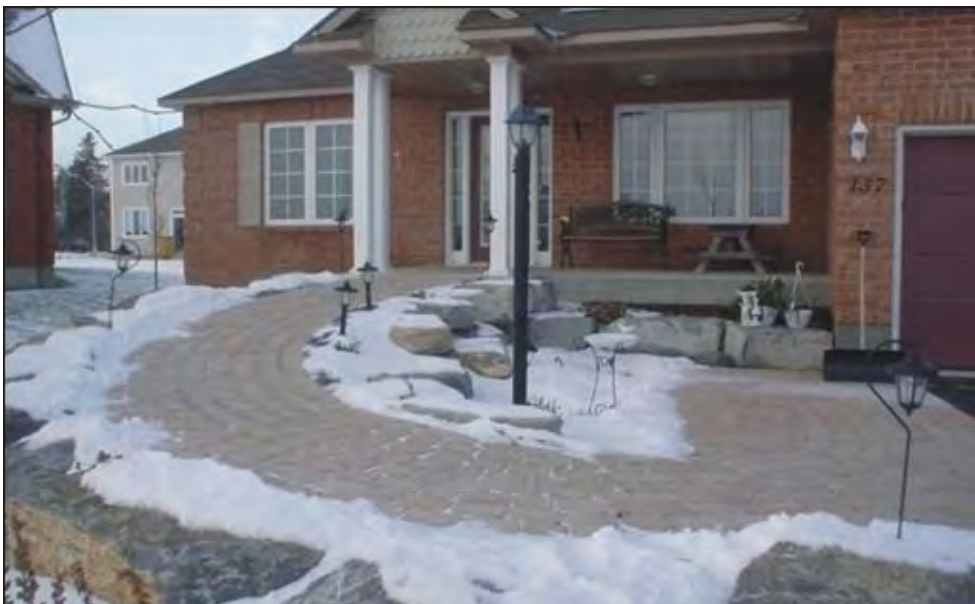
■ RAMP that doesn't look like a ramp works not only for people with disabilities. It makes life easier for everyone.
