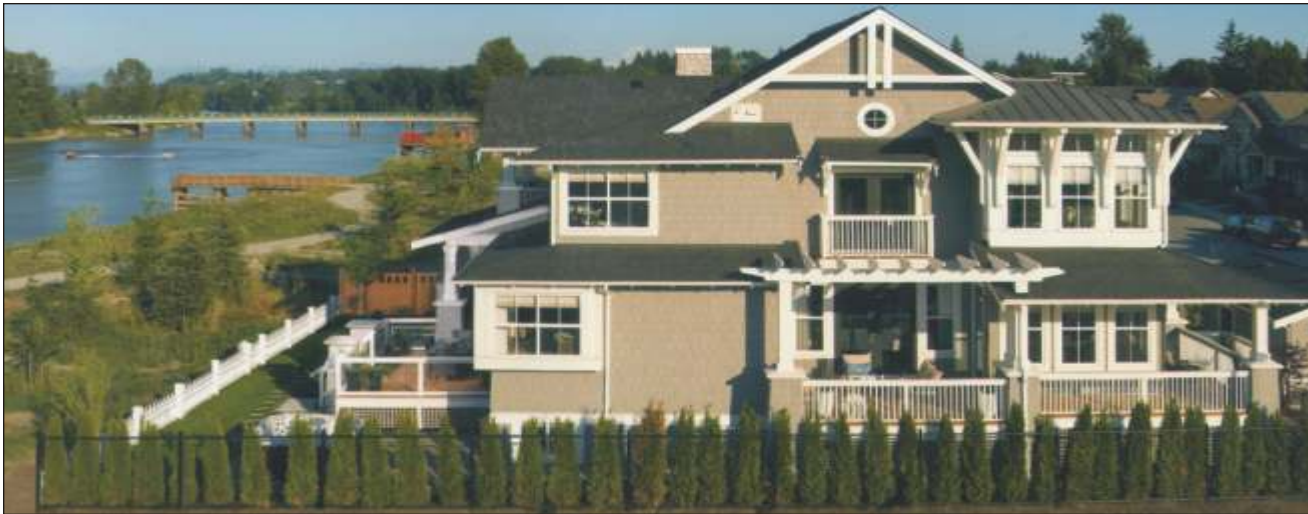
■ A STRIKING exterior inspired by a blend of Cape Cod and Craftsman architecture are key features of Headwater , Bedford Landing which won the SAM Award for Best Single-detached Home of more than 2,200 square feet for Vancouver's ParkLane Homes Ltd.
